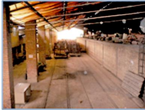
Figure 2. Tunnel kiln installed as the project in Las Tapias 3 Ceramic.
