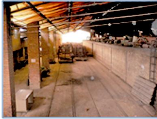
Figure 2. Tunnel kiln installed as the project in Ceramic Las Tapias 3.
